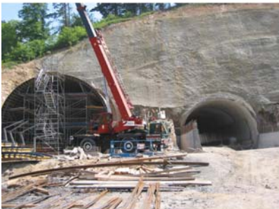
Tunnelling demands a detailed geological knowledge of underground materials.
