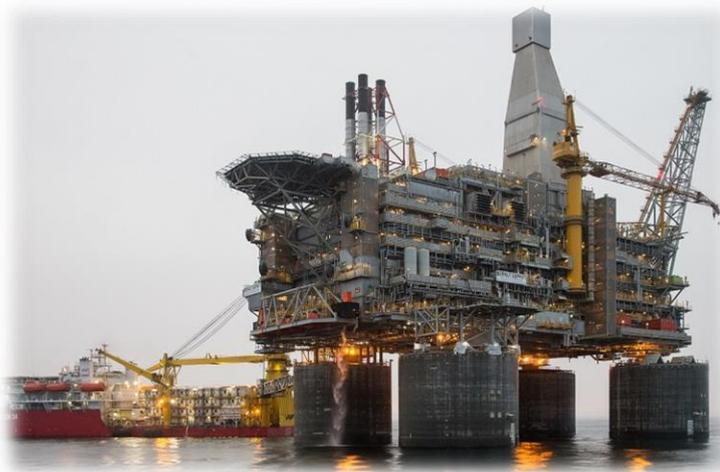
Figura 3.5: Gravity Base Structure
