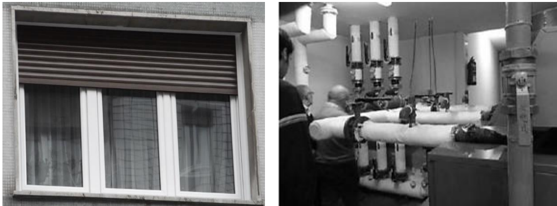
Figure 52 Reforms carried out: improve windows properties (a) and replacement of the heating generation centralized system (b)
