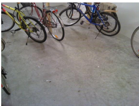
Figure 13: The real floor of the bicycle room
