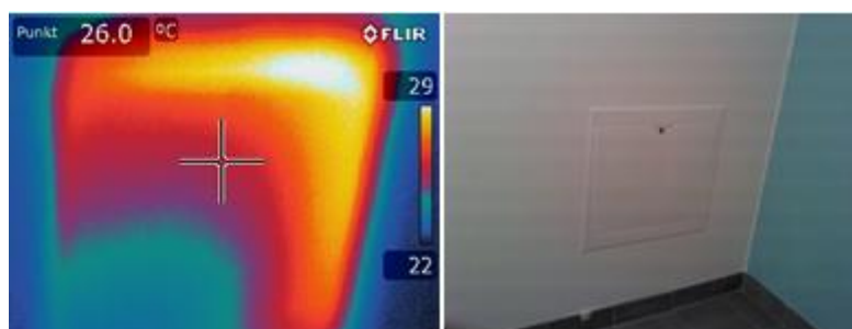
Figure 16: The water measuring box when is closed
