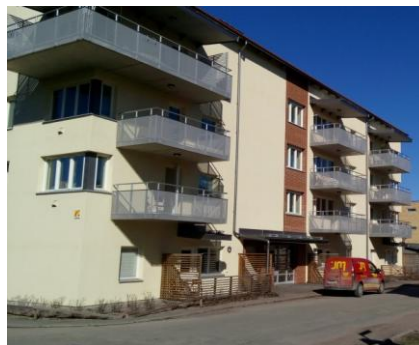
Figure 20: The brick and the concrete walls
