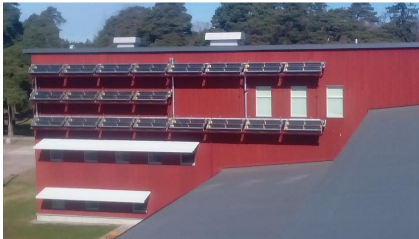
Figure 4.1. C-PVT collector's installation at HiG
