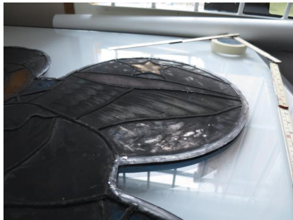
Figure 7: example of degradation in a stained glass window at Uppsala Cathedral.
