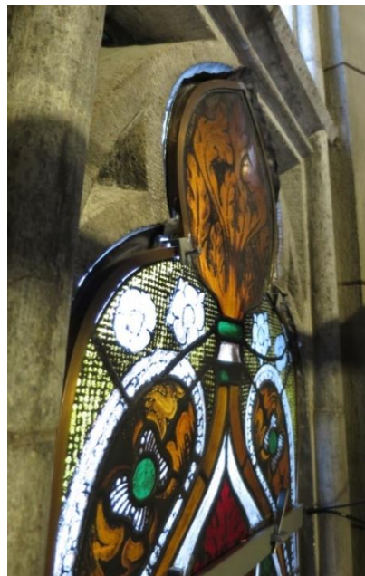
Figure 3: detail of the top slot in one of the stained glass window panes.
