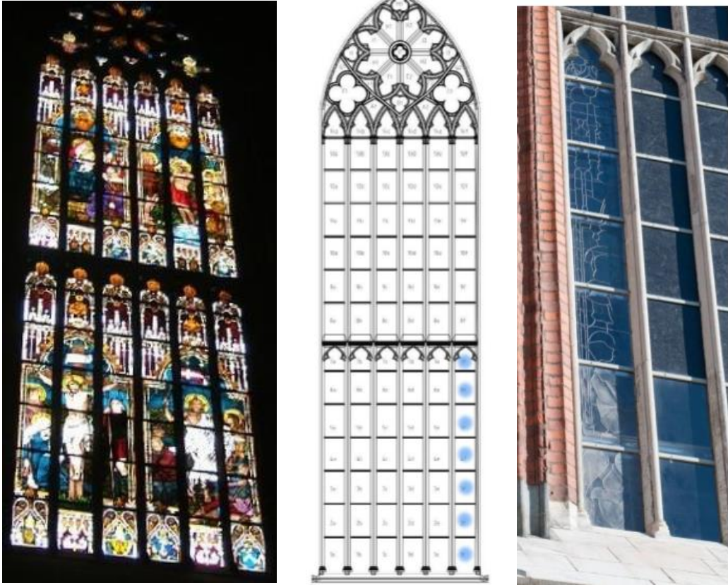
Figure 2: Sonens fönster (a) view of the stained glass from the inside, (b) scheme of the stained glass, (c) view of the window from the outside.
