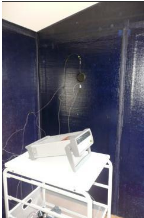
Figure 4.29.- Mock-up interior after sandwich panel installation.
