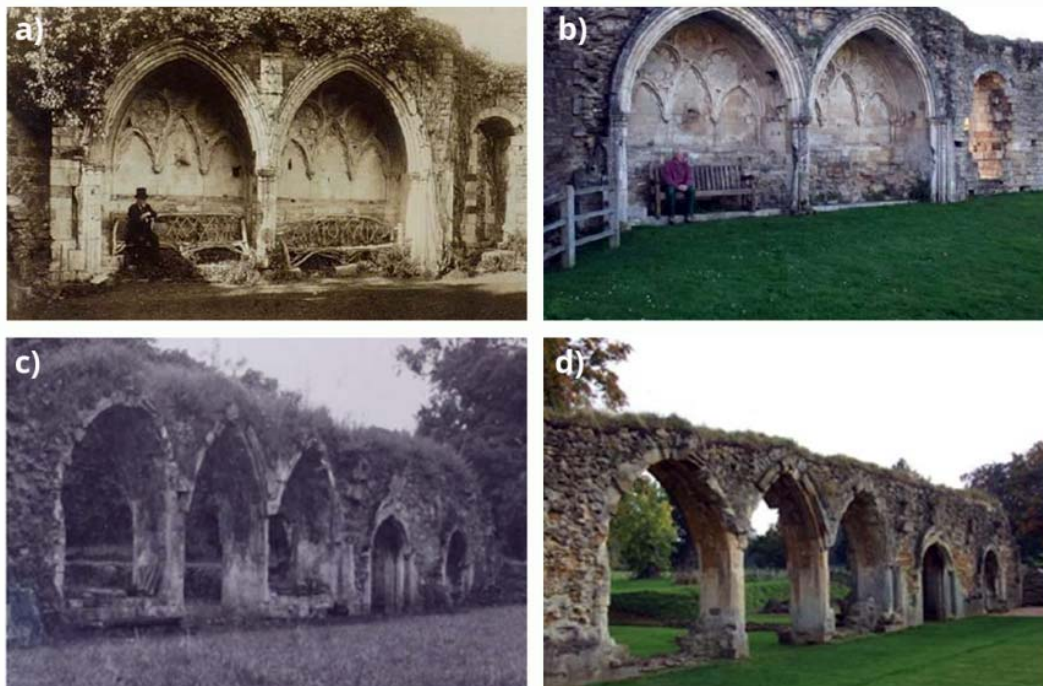
Figure 7.4. Images of ruins historical monuments of England, in which their past and present state can be compared. a-b) Kirkham Priory (19 th image vs 2007) where past conservation methods led to removal of the protective vegetation cover. c-d) Hailes abbey (1937 vs 2007), where an alternative green method was applied 10 .
