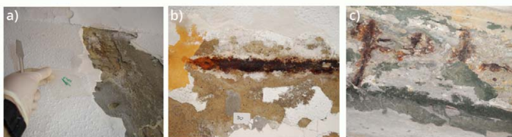
Figure 6.8. Selected photographs of the affection observed in the stairs area. a) Salt efflorescences and detachment of the plaster of the wall. b-c) Wet structures covered by efflorescences.
