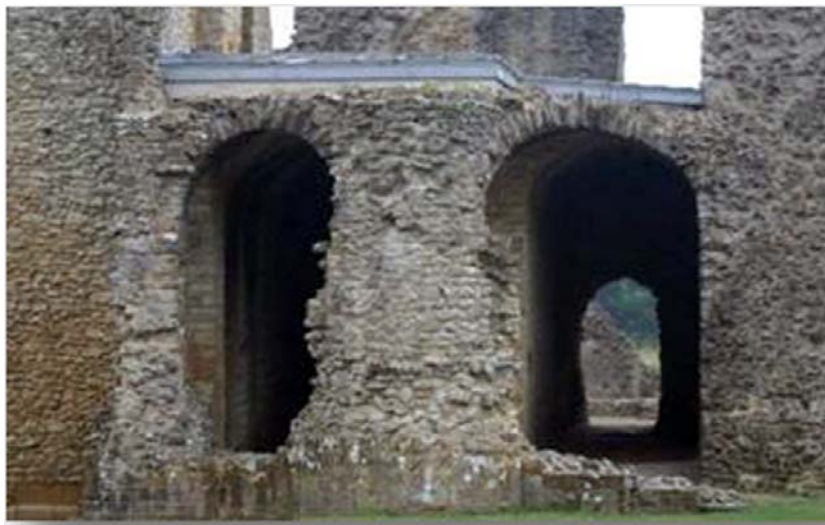
Figure 7.2. Images of a ruin historical monument of England, in which the Hard capping method was applied.
