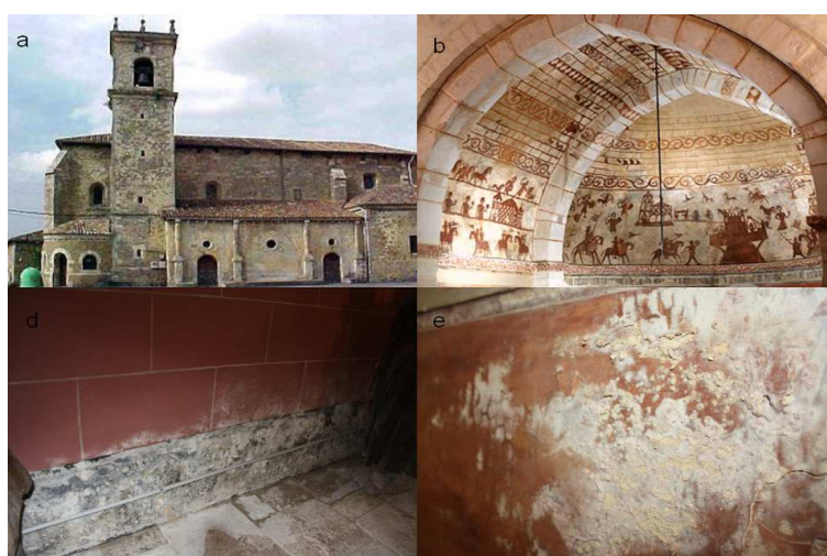
Figure 1. a) External view of the Assumptions' Church, b) Romanic mural paintings found inside, d) and e) Efflorescence salts analyzed with the handheld device.
