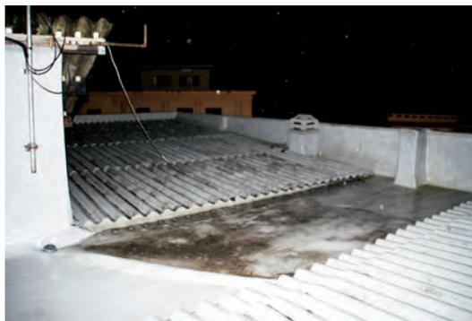
FIGURA 5. 89. KALE NAGUSIA 2, CUBIERTA PLANA CON PLACAS DE FIBROCEMENTO
