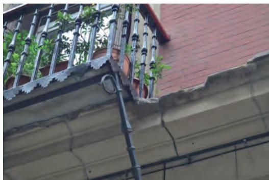
FIGURA 5. 64. KALE NAGUSIA 15, VUELO EN CORNISA CON ESTRUCTURA METÁLICA Y LOSA DE PIEDRA
