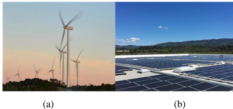
Figure 2.2(a) The wind generation park constructed in Chile by Gamesa[15] and (b) the solar system installed in California and developed by General Electric.
