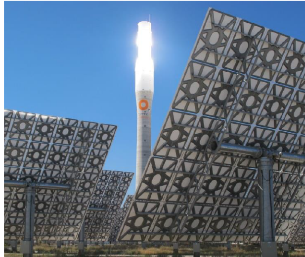
Figure 1. GEMASOLAR Power Plant, Torresol Energy property, © Torresol Energy.
