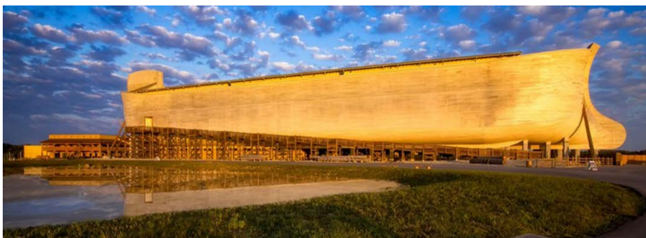
Figure I-27 Acetylated wood used in a civil engineering project (Accoya ® ), Cincinnati (USA), 2016.
