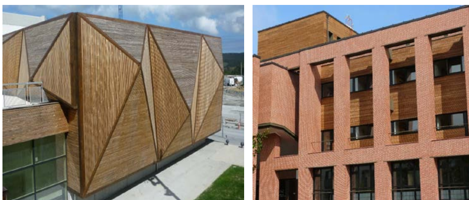
Figure I-30 Thermally modified façades, Leioa and San Sebastian, Spain.
