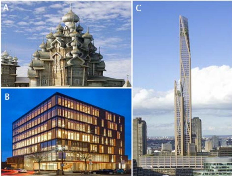
Figure I-31 Examples of tall wood buildings: (A) Kizhi Pogost-37.5m, Russia, 1862; (B) WIDC-30m, Vancouver, Canada, 2014; (C) Oakwood tower-300m, London, conceptual stage.
