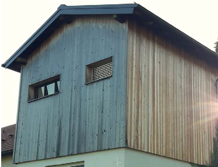
Figure I-13 Wood color changes by UV degradation (Kulch, Austria).
