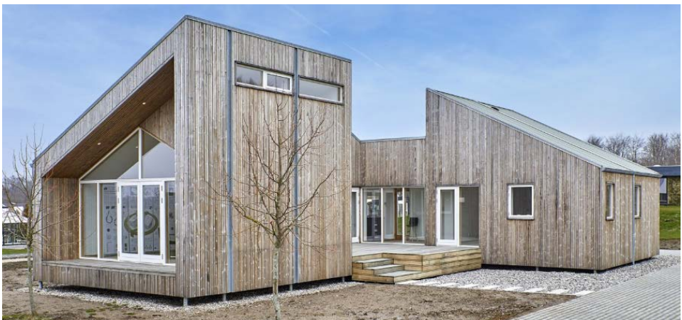
Figure I-29 The Biological House, Middelfart (Denmark), using Kebony® for the exterior cladding.
