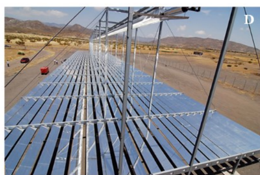
Figure 1-2. A) Tower power. Gemaspower plant in Andalusia, Spain (Torresol Energy) [5]. B) Parabolic dish (DLR, Markus Steur) [5]. C) Solar receiver for trough technology (Ultimate Trough® test loop installation, California) with permission from schlaich bergemann partner. D) Solar receiver for Linear Fresnel technology (Plataforma Solar de Almería (PSA) [6].
