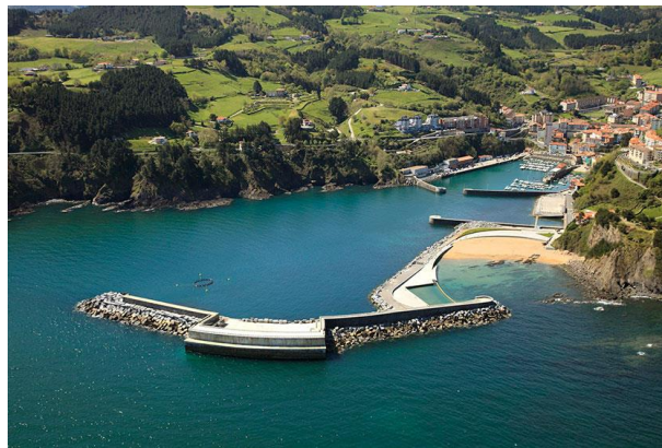
Figure 1. View of the Mutriku Wave Power Plant built at Atlantic coast of the Basque Country [EVE].
