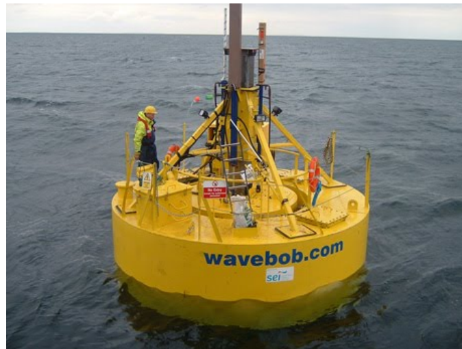
Figura 9-7: Boya Wavebob instalada en Irlanda (OffshoreWind, 2013)
