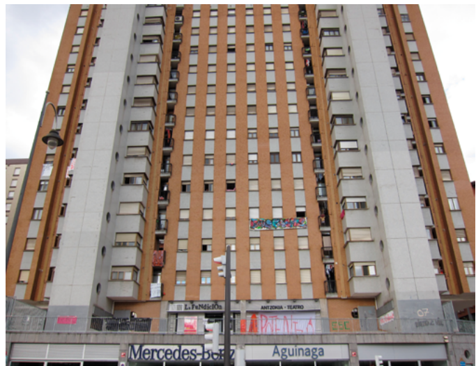
Figure 2.19. Residential building where La Fundición is located, showing some of the placards of the project Your cheer up message here , 2013.
