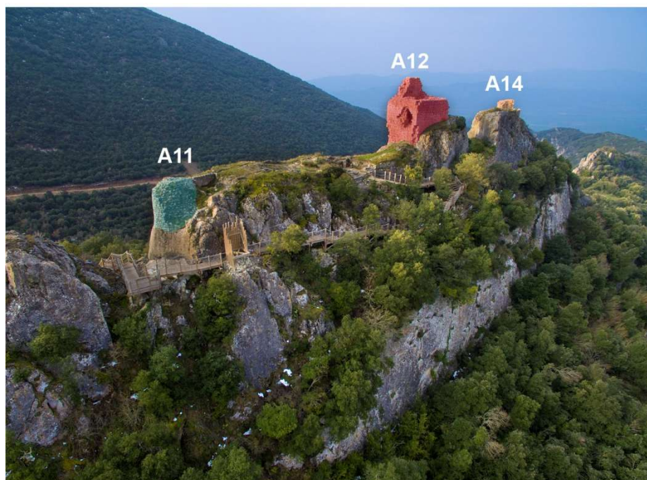
Figure 2. Studied structures at Portilla Castle. West Tower (A14), Tower Keep (A12), and East Tower (A11).
