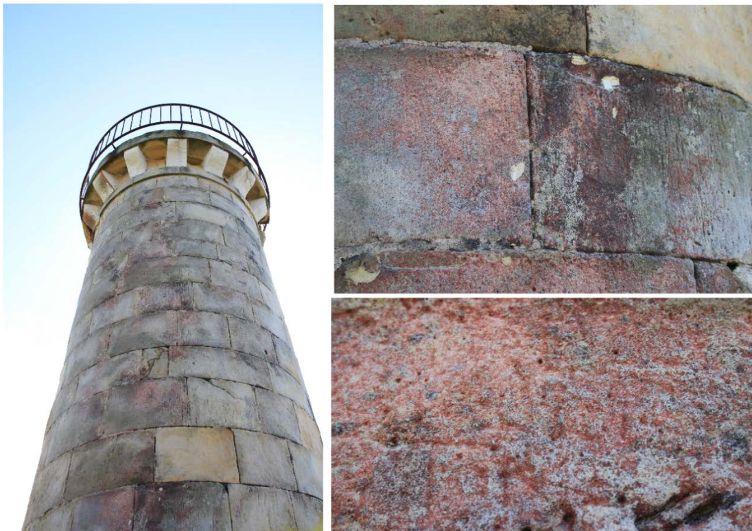
Figure 1.4. Trentepohlia algae colonization affecting the tower of La Galea fortress, a fortification from the 18 th century (Getxo, Basque Country, Spain).
