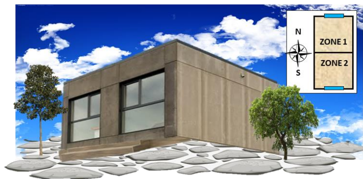
Figure B. 2 Picture of the case study building
