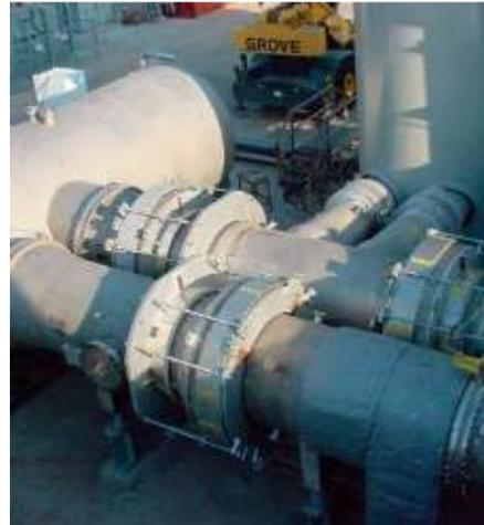
The intercooling system takes compressed air from the low-pressure compressor, cools it to optimal temperatures and then redelivers it to the high-pressure compressor. In providing a constant stream of low temperature air to the high pressure compressor, the work of compression is reduced. The result is a higher pressure ratio (42:1) and increased mass flow (500 lb/sec).
