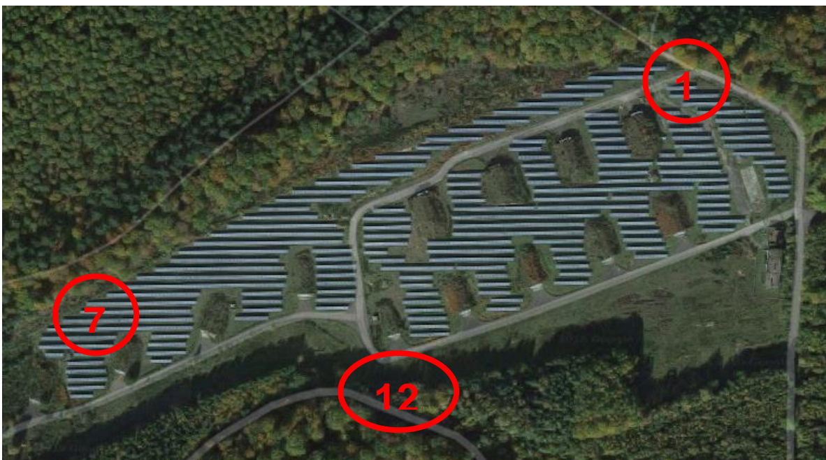
Fig 1.1: Bird's eye view from the 3 MW Photovoltaic power plant.
