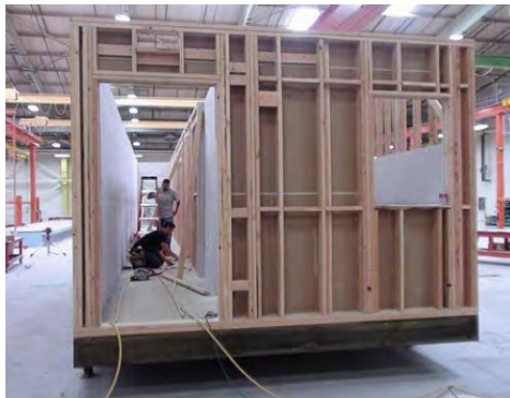
Figure 3.1.1 Load bearing module made of
