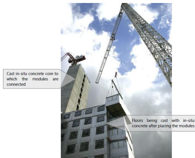
Figure 3.2.2 Image of a building with this system.
