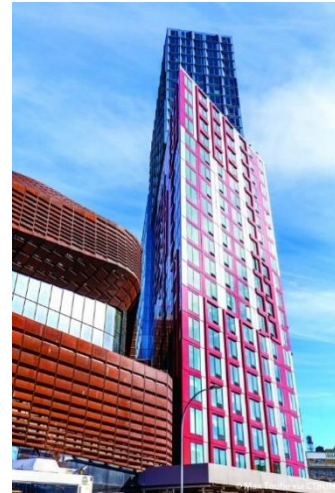
Figure 7.4.1 Actual image of the building.
