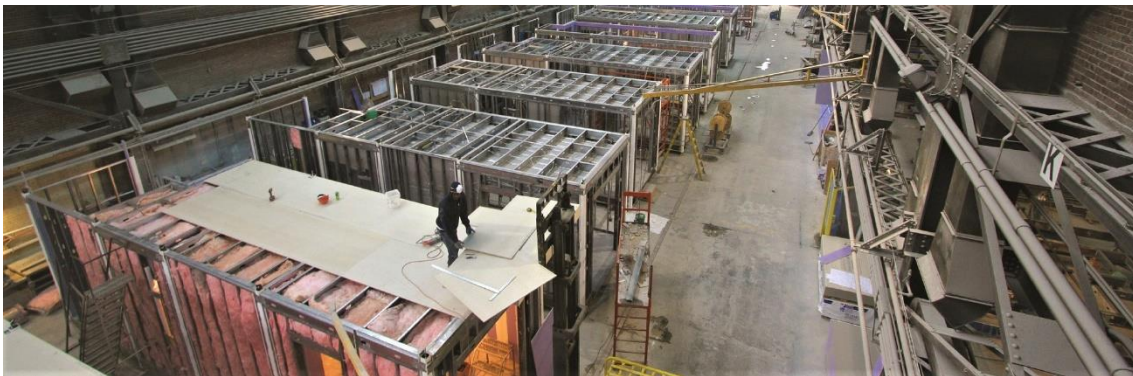
Figure 2.2.3 Image of a manufacturing plant, where the finishes are being done.
