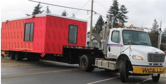
Figure 2.2.5 Transport of a modular unit.
