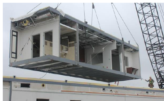
Figure 3.1.2 Steel corner supported module.
