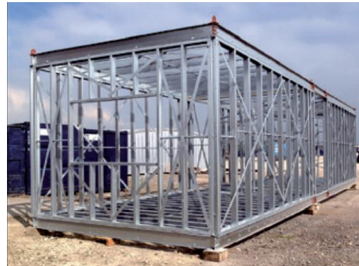
Figure 2.3.3 Light steel frame modular unit
