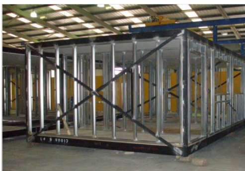
Figure 3.1.3 Light steel corner supported module
