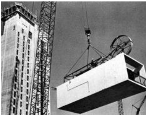
Figure 2.1.4 Craning operation in Hotel Palacio Del Rio, San Antonio, U.S.A.
