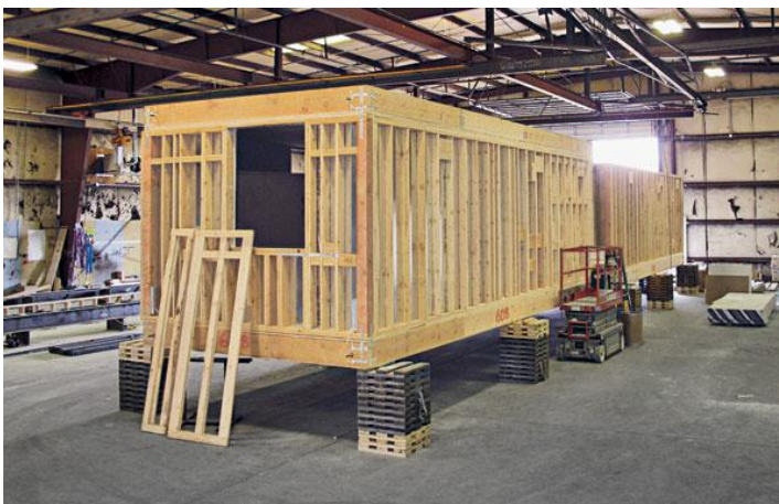
Figure 2.3.1 Wood made modular unit at the manufacturing plant.
