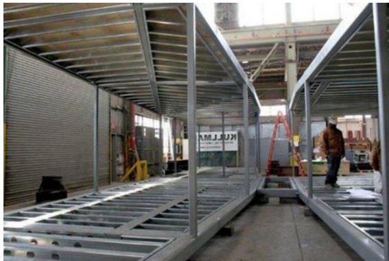
Figure 2.3.2 Corner supported steel module
