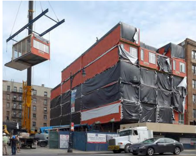
Figure 7.1.1 Assembling process of units.
