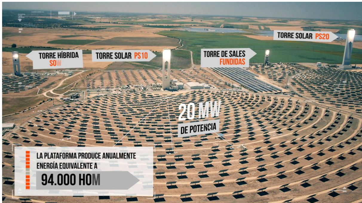
FIGURA 21: TORRE CENTRAL PS10, ABENGOA (MICROGAL TV)
