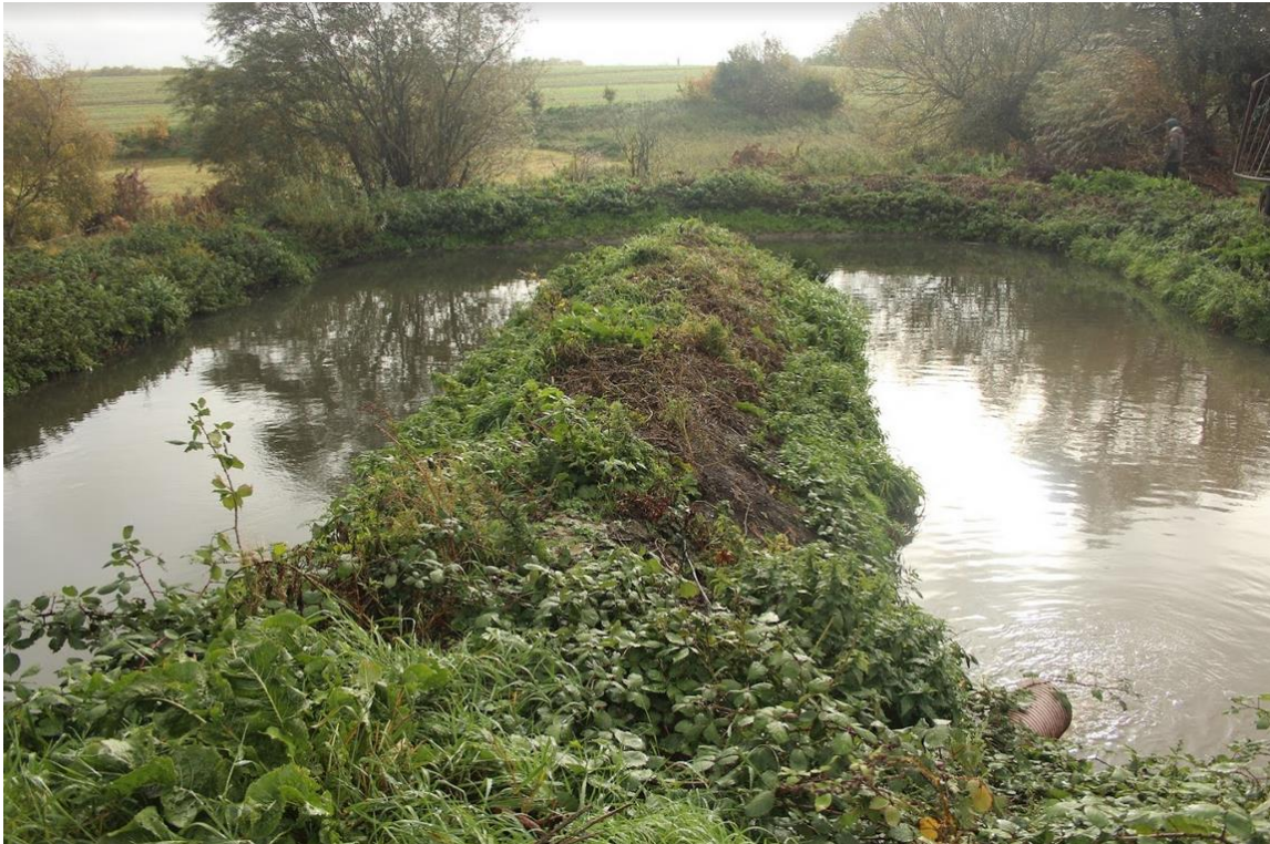
Figure I. 6. Picture of basin BLB0140 at Damvej in Blegind. In the bottom right corner, the inlet is visible. The outflow pipe is not visible on the picture; it is located in the bottom left corner
