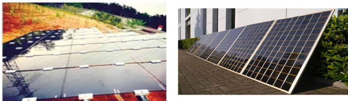
Figure 20. Left: Power plant composed of 32 modules with an area of 45 \times 65 \text{ cm}^2 connected in between. [109] Right: 7 \text{ m}^2 printable perovskite-based panels. [110]
