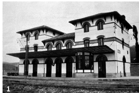
Figure 4.80 Railway station area of Maeztu composed of loading bay and passenger building (left). Alejandro Mendizábal, FEVE's Collection in RMA
