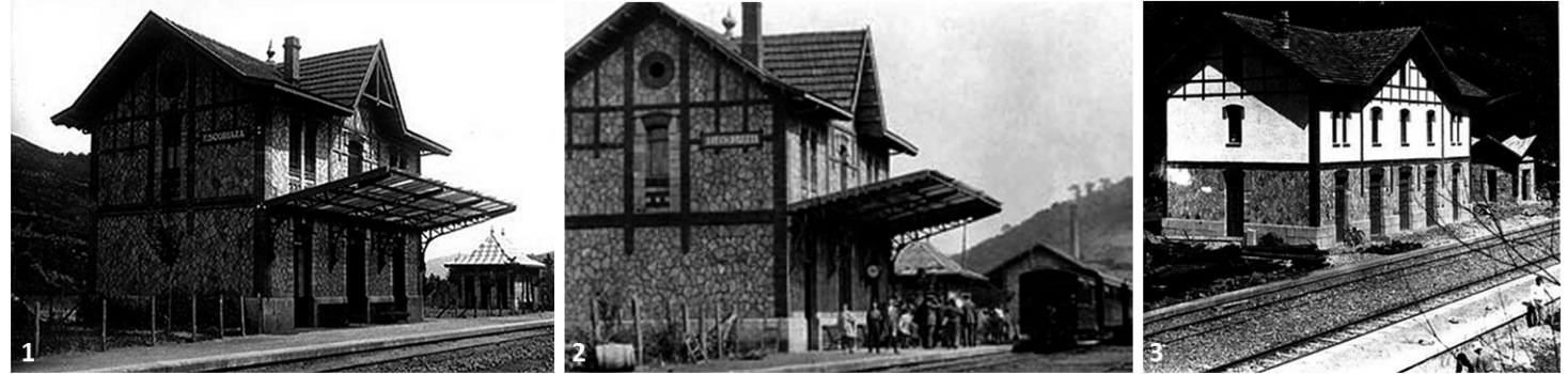
Figure 4.63 Railway station area of Antoñana composed of loading bay, passenger building and electrical subcentral (left). Alejandro Mendizábal, FEVE's Collection in RMA
