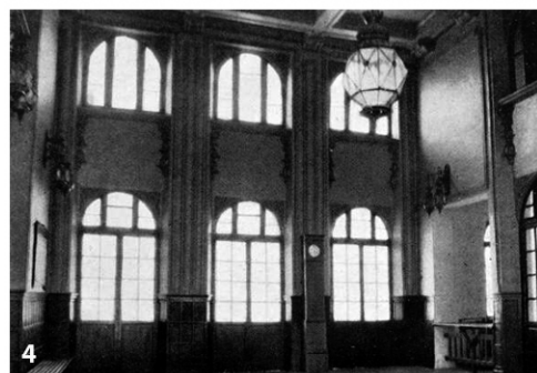
Figure 4.82 Passenger building of the railway station of Maeztu (2). Idem
