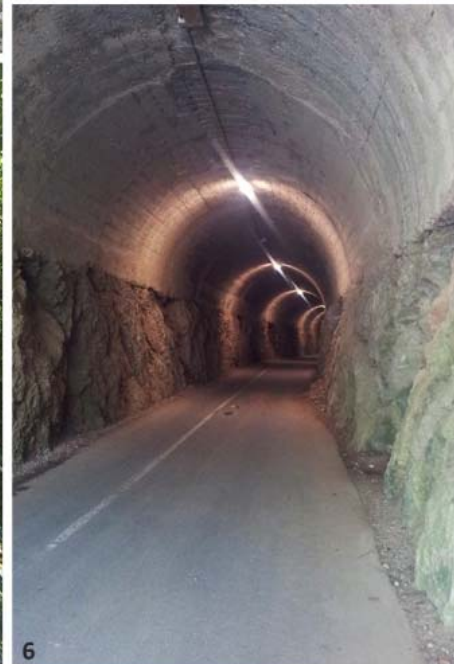
Figure 4.158 Artificial tunnel of Fuenfria (1)
