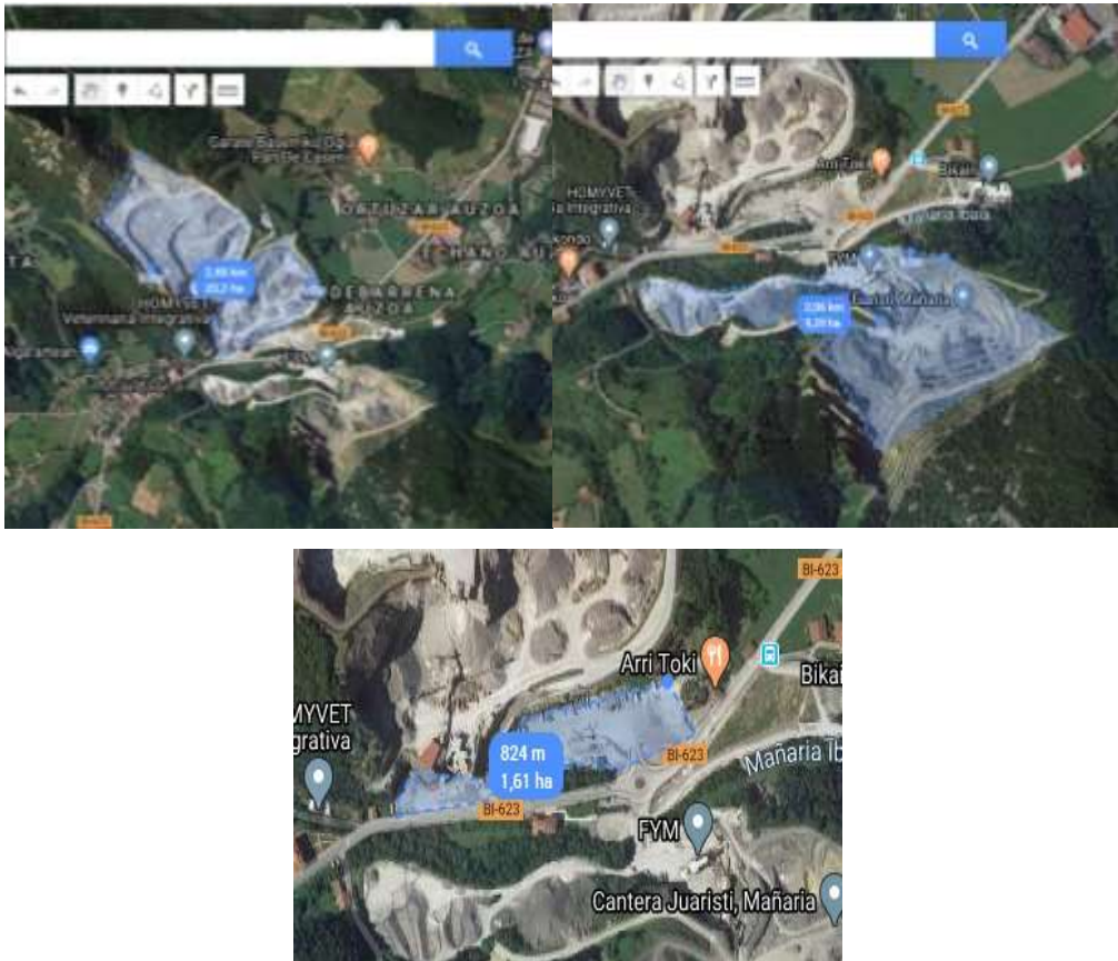
Fig. A2.2. Extension of the AMANTEGUI facilities. Screenshot of the satellite map of Google.
