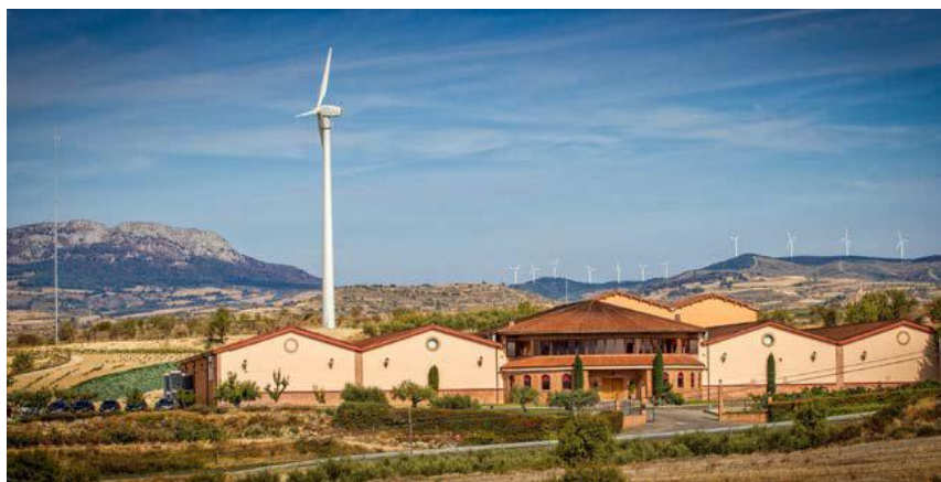
Figure 1. Horizontal axis wind turbine in Pierola wine cellar (Moreda, Araba)
