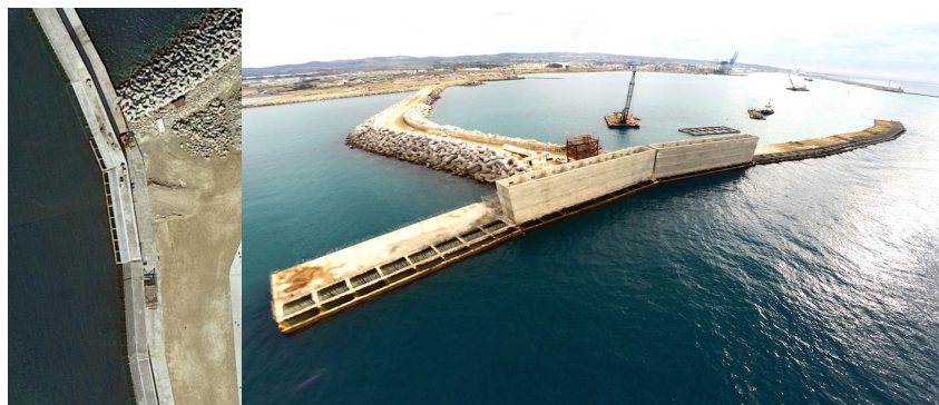
Fig. 2.26: The caissons of the REWEC3 in the port of Rome, photo credit duomi.it
