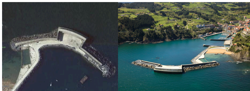
Fig. 2.25: Aerial view of the Mutriku Wave power plant, courtesy of EVE
