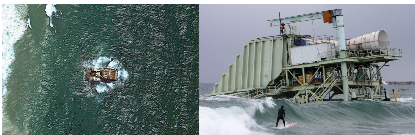
Fig. 2.23: The wrecked Oceanlinx off Port Kembla from [Joh15]
