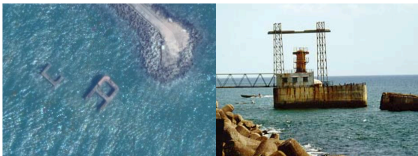
Fig. 2.19: Vizhinjam near-shore OWC plant from [The05]
