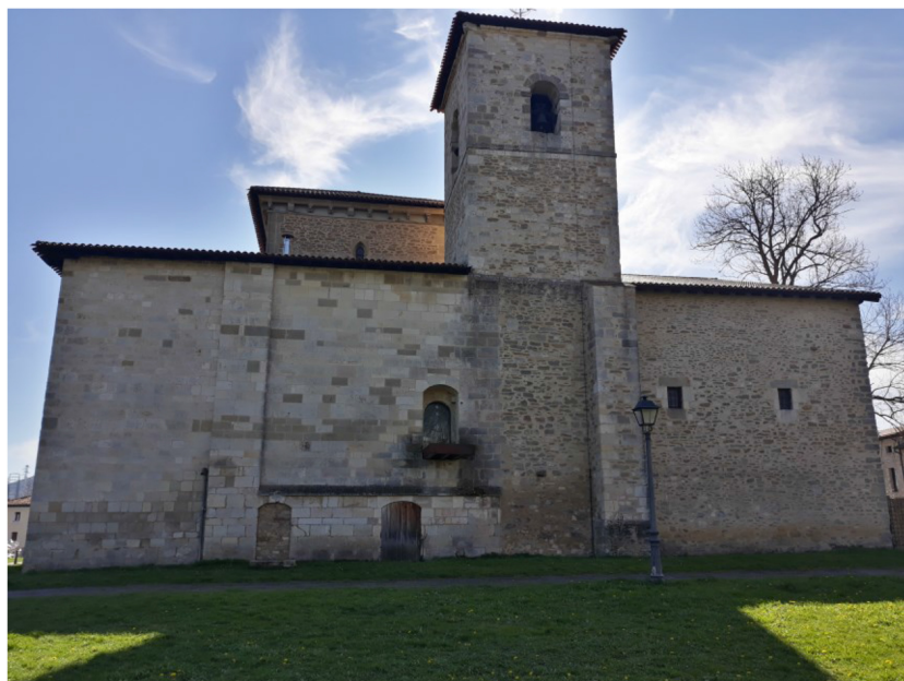
Fig. 3. North elevation of the Basilica of San Prudencio de Armentia. The left part is made using ashlars, while the right part corresponds to rough ashlars.
