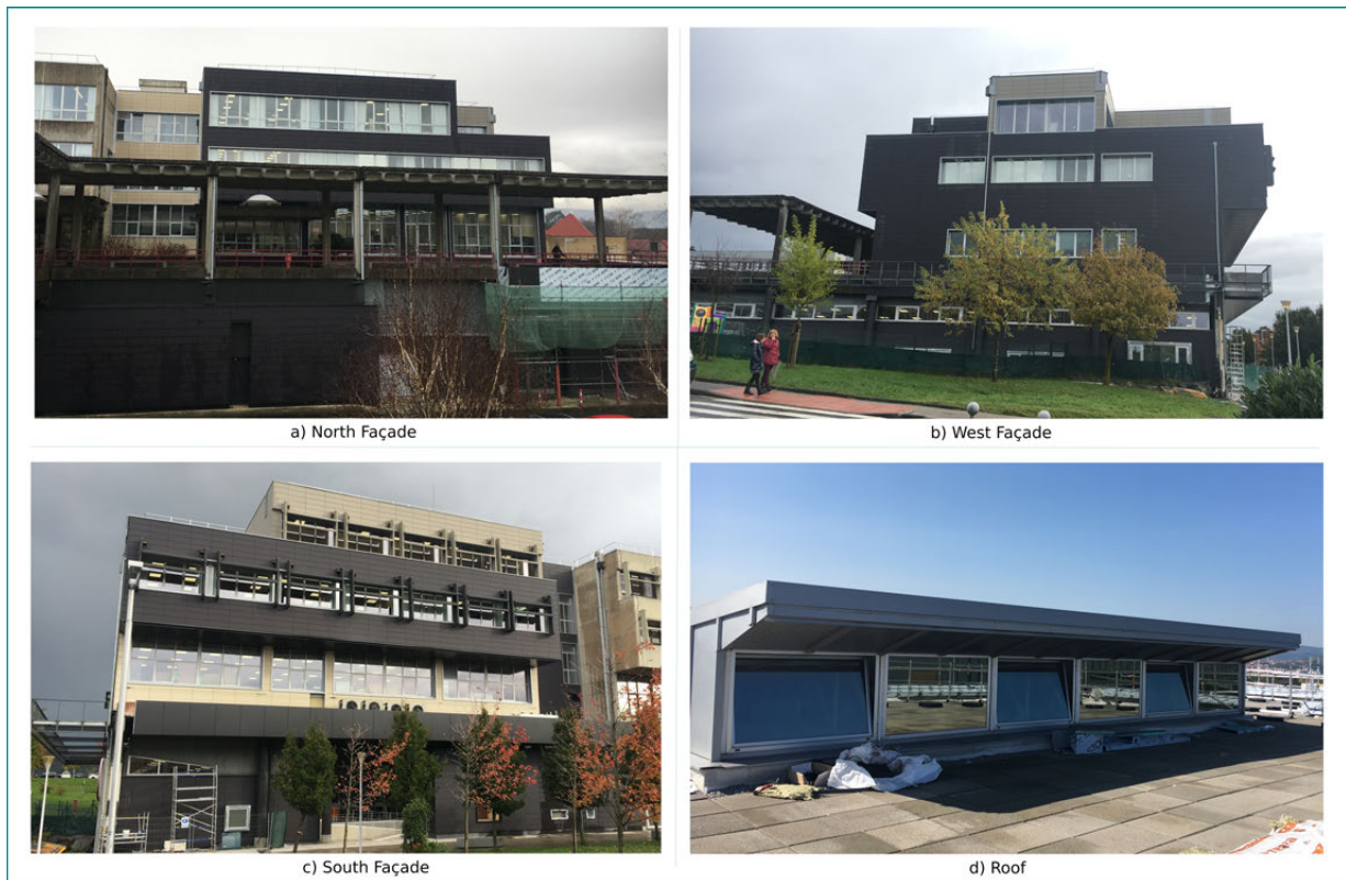
Figure 4.2: The UPV/EHU administrative building in Leioa post-retrofitting: a) northern façade, b) West Façade, c) southern façade, d) Roof.
