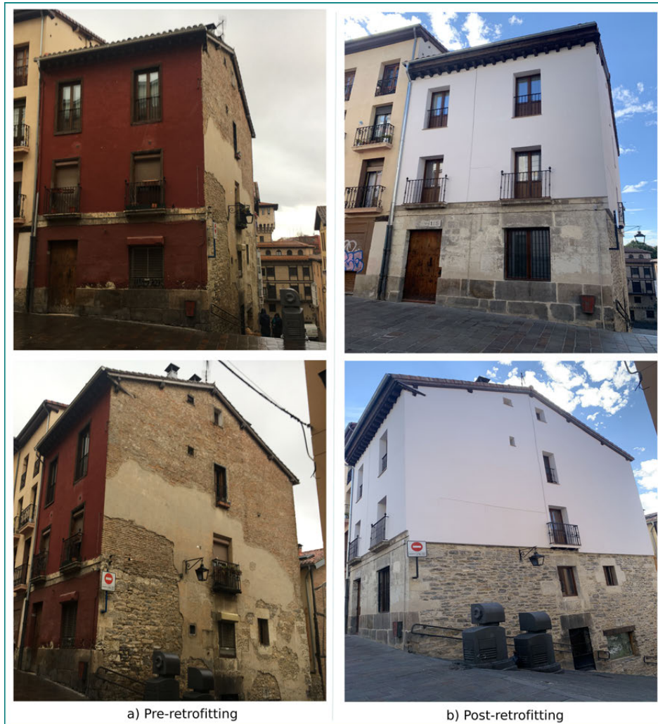
Figure 4.26: The residential building in Vitoria-Gasteiz: a) Pre-retrofitting, b) Post-retrofitting.
