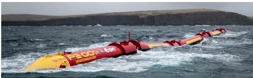
Figure 3 Pelamis Wave power P2-001 device installed. Courtesy of EMEC [26]
