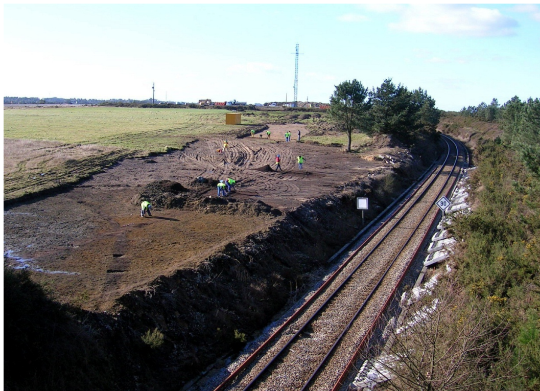
Figure 8. Panoramic view of the area once manual excavation work had begun.
