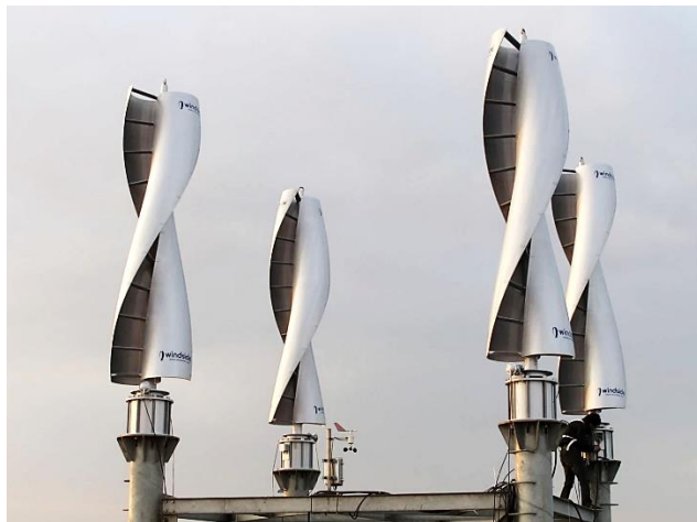
Figure 19. Savonius wind turbine [Source: [33]]
