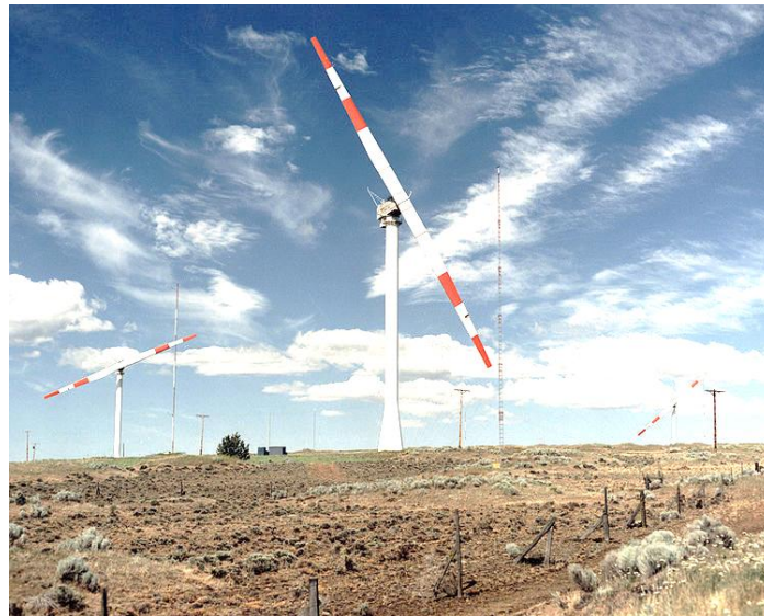
Figure 16. Two-bladed wind turbine [Source: [30]]
