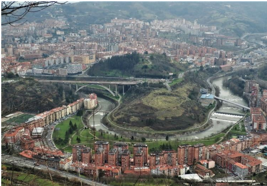
Figure 27. Picture of a possible location of the wind turbines. [Source: [43]]
