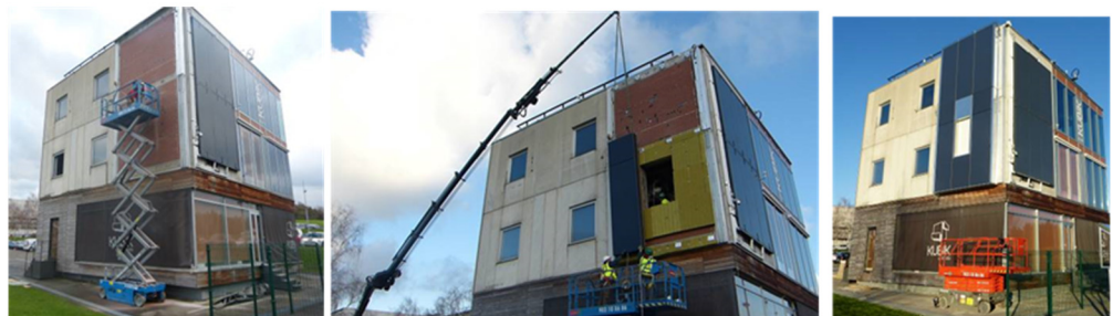
Figure 12. Installation of the plug and play façade system.
