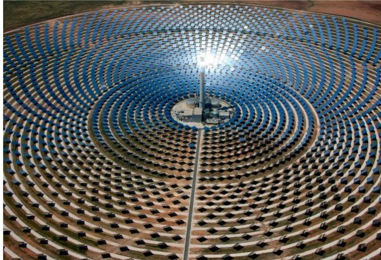
Figura 2.3 Central de campo circular Gemasolar (Torresolenergy, 2020)
