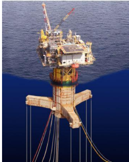
Figure 2-10. Chevron USA Typhoon SeaStar-profile TLP for offshore Oil&Gas production. Source: Matten (2002) 21
