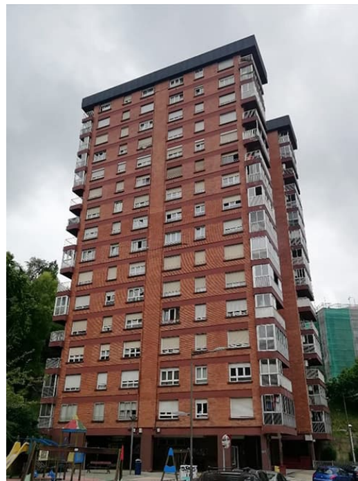
Figure 3. Building at Bertsolari Txirrita, 38, in San Sebastián.
