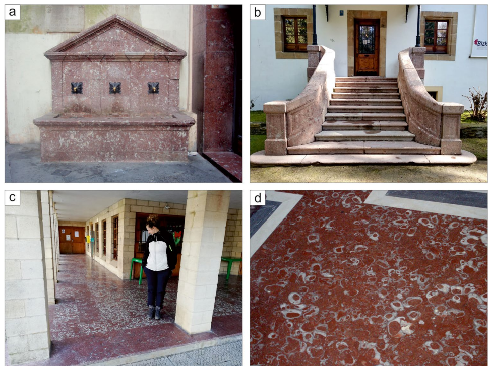
Fig. 3 a Fountain in Iturribide Street in Bilbao (Bizkaia, Spain) from 1894. b Stairs of the Euskal Herria Museum in Gernika (Bizkaia, Spain). c Floor tiles on the outside of the Ispaster pelota court (Bizkaia, Spain). d Red Ereño tiles at the entrance of St. Peter's Basilica in the Vatican (Italy)
