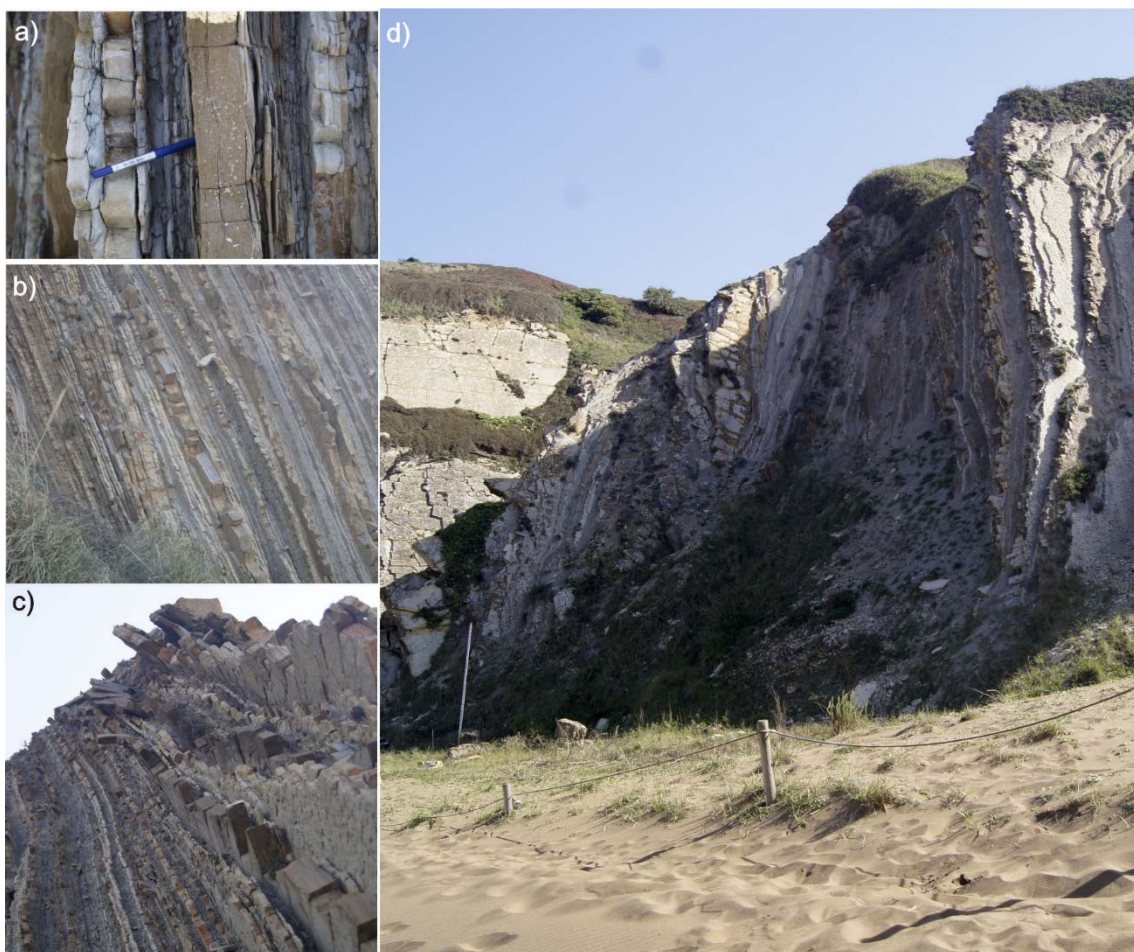
Fig. 5. Rock mass and instability processes characterization. a) Flyschoid sequence; b) planar instabilities on the main slope on J_1 ; c) block toppling on the secondary slope over J_2 ; d) maximum runouts at the northern end of the protected dunes area.
