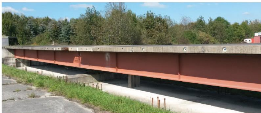
Figure 2. UniBw bridge (Benndorf et al., 2016)
