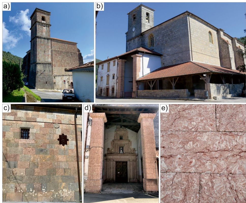
Fig. 5 a San Miguel Church in Ereño (Basque Country, Spain). b Andra Mari Church in Gautegiz-Arteaga (Basque Country, Spain). c Detail of the dimensions of stones of different tones of San Miguel Church (ashlar width varies between 0.5 and 1 m). d Pilasters from the main door of Andra Mari Church. e Detail of the ashlar blocks containing polyconitid rudists (block width is 1 m)
