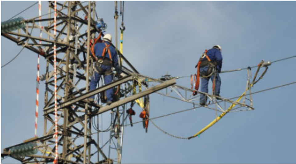
Fig. 5. Sagging the gap-type conductor
