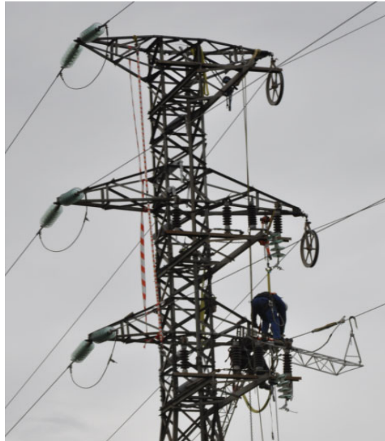
Fig. 1. Stringing the gap-type conductor
