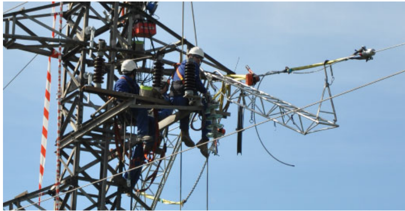
Fig. 4. Pre-sagging: pulling the new conductor by an aluminum gripping clamp
