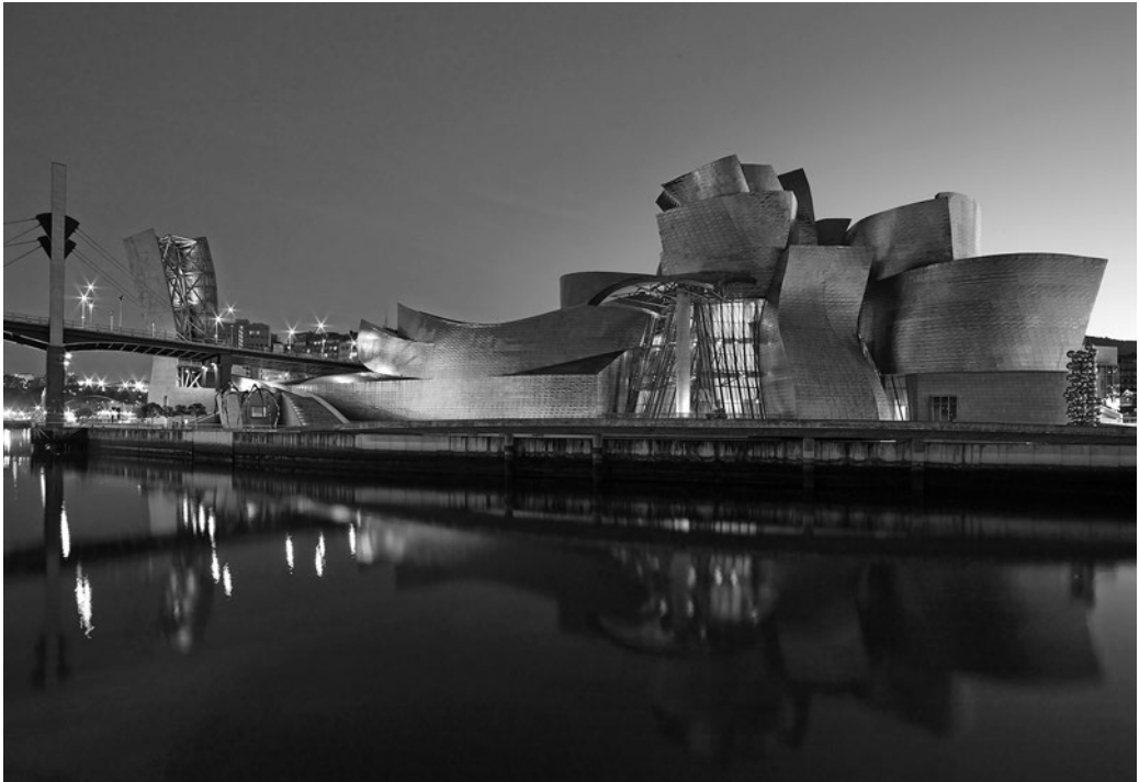
Figure 8.5 Guggenheim Museum Bilbao Source: Courtesy of FMGB, Guggenheim Bilbao Museoa, 2015.
