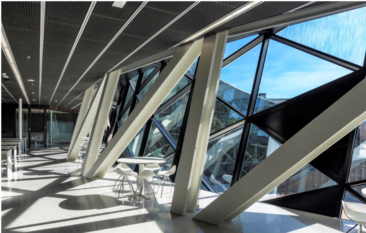
Figure 7. Inner view of the south facing circulation gallery where different elements of the curtain wall can be observed.
