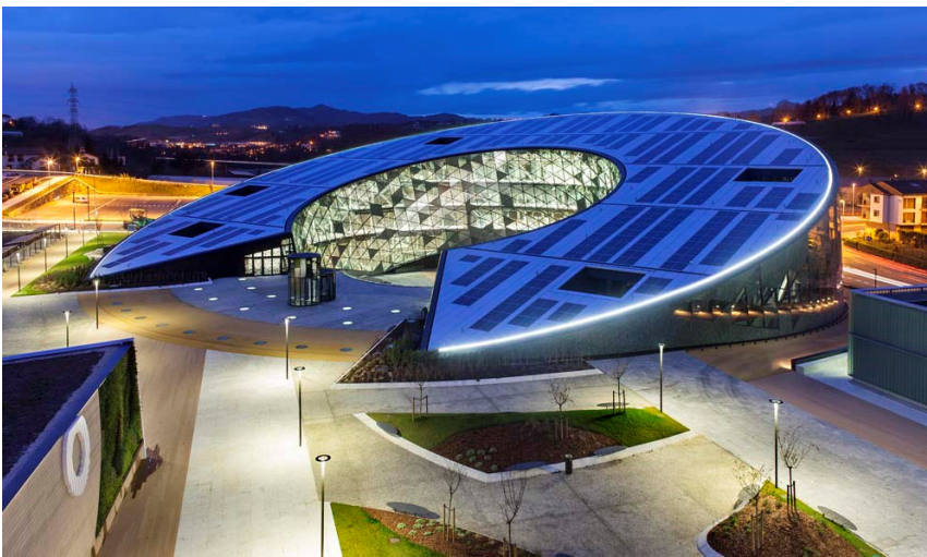
Figure 3. Inclined PV roof of the Zero building.
