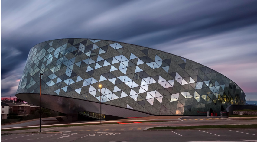
Figure 2. Front façade of the Zero building.
