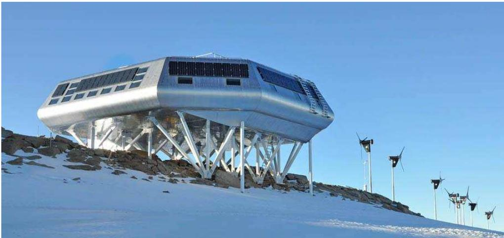
Figure 9: Antarctic Princess Elisabeth Research Station is electrically fed by means of an islanded microgrid based on renewable energies. *Courtesy of Antarctic Princess Elisabeth Research Station.*
