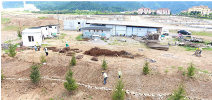
Figure 7. Construction process, (Düzce Umut Atölyesi, 2017)
