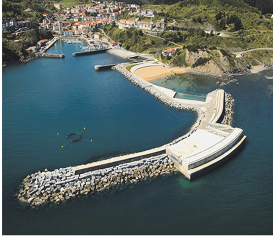
FIGURE 1: The OWC power plant of Mutriku.
