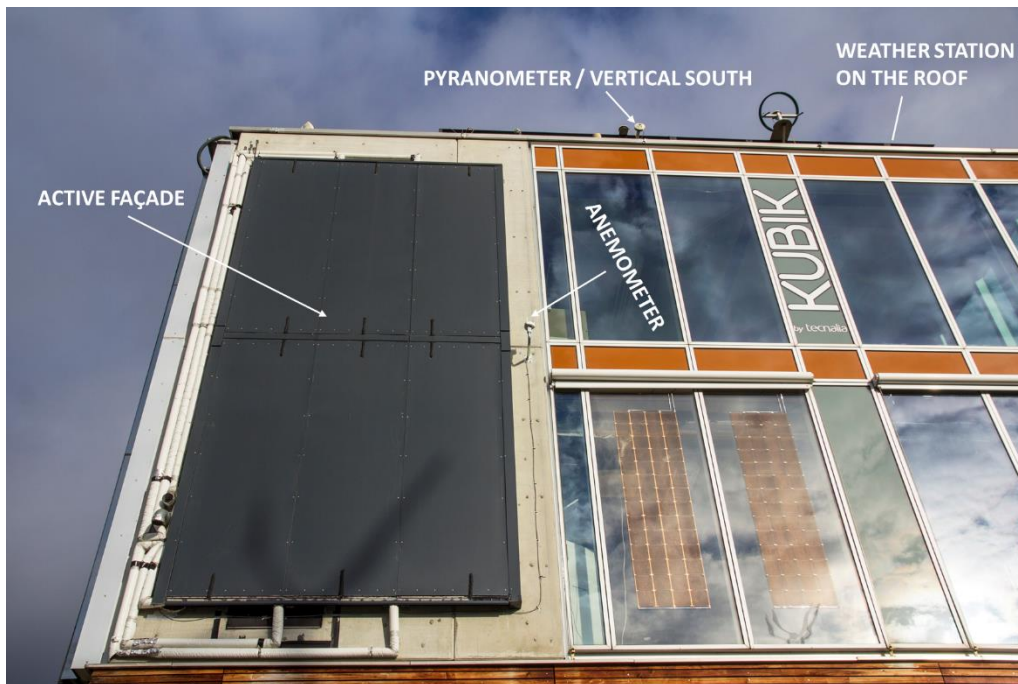
364 Figure 8: Panels installed in the south façade of Kubik® building
